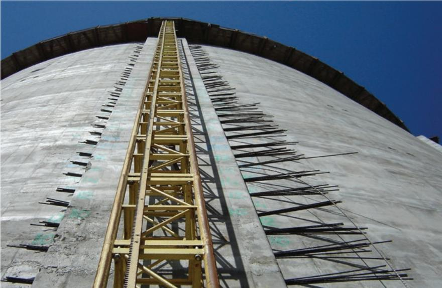
Post-tensioning increases structural resilience while allowing reduced wall thickness, and reducing crack widths. Minimal permeability and high levels of corrosion protection are also required for all LNG/LPG structures; the post-tensioning system must therefore be designed and installed under strict quality controls, with materials and processes meeting specific certification and performance requirements.
