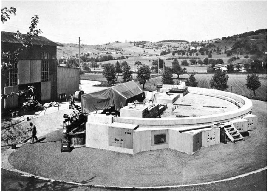
Full-scale installation and tendon replacement test with tendons consisting of strand and wire tendons.
