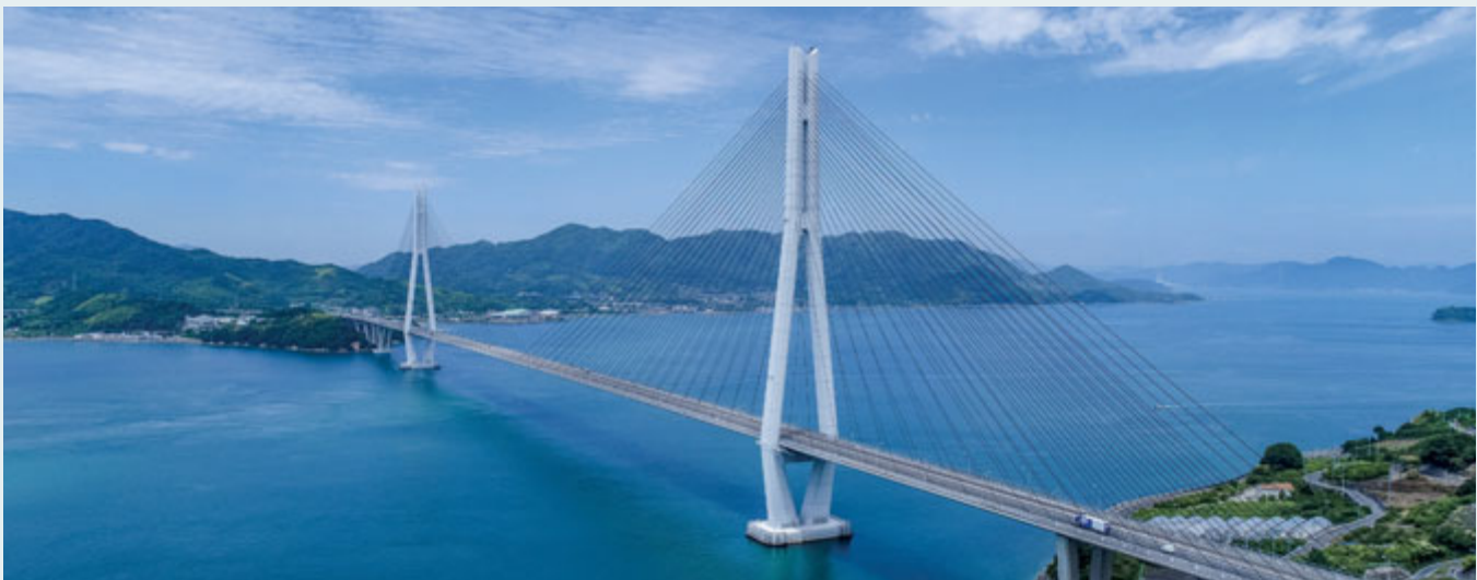
Tatara bridge, Japan.
