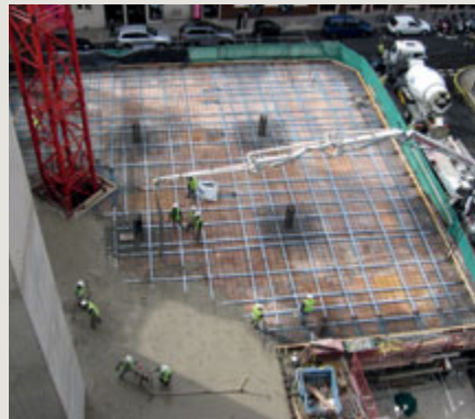
Crown House, London. A 12-story office block, behind a retained Victorian façade. PSC reduced concrete quantity requirements, thinning the floor slabs with bonded flat slab tendons. The increased spans gave the owners greater flexibility and space.
