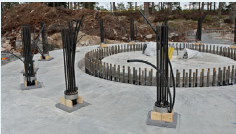
The foundations are secured using ground anchors.
