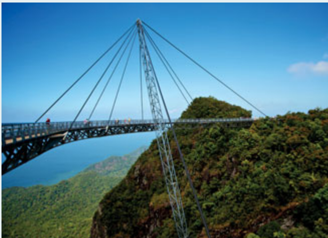
Machinchang Bridge, Langkawi Island, Malaysia.
